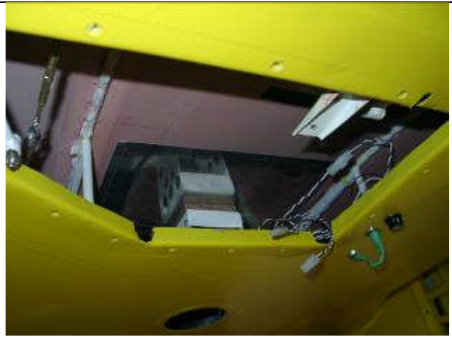
Newly installed ground plane
