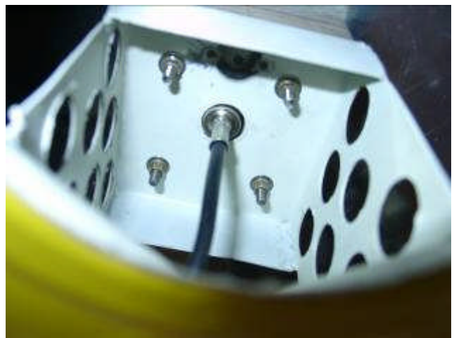
Newly installed BNC connector on Comm 1 antenna. Because of the differences in the mounting method, the BNC connector is buried in the SOCOW and is only accessible after removing the antenna from the fuselage. The nuts shown here took about an hour to install because of limited accessibility. Later they would be replaced with an aluminum sheet with four nutplates.
