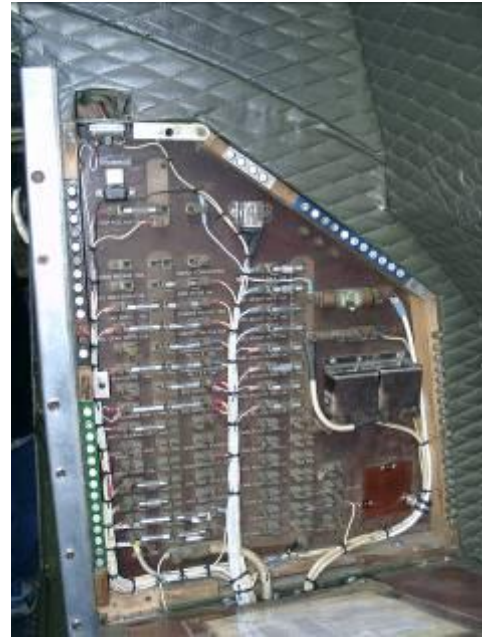
Fuse panel on left side rear cockpit wall. Note spare fuses stored in the wood frame around the box.
