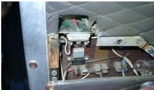
Bomb bay light switch immediately above fuse panel
