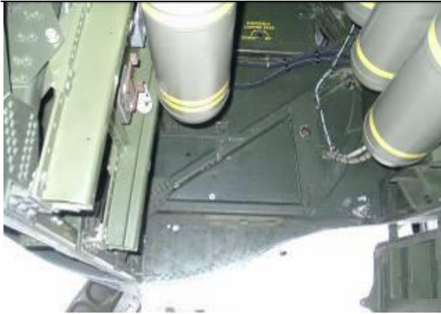
View of main wing spar truss at the front end of the bomb bay. Near the top of the picture is the hole to insert the crank to manually lower the landing gear.
