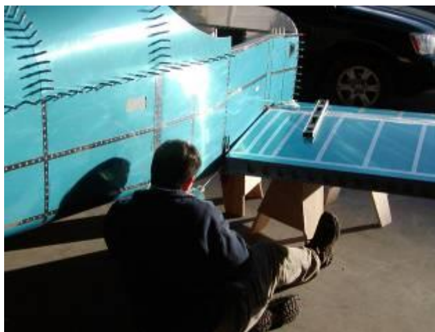
Jim at a high pucker factor moment – drilling the rear spar attachment
